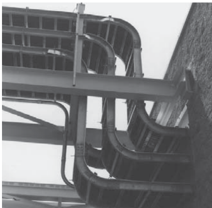
Figure 5-20. Cable trays are used to support cables in industrial settings. (PW Industries, Inc.)
