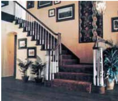
Figure 18-9. This L-shaped stairs is wide enough for moving furniture up and down. (C-E Morgan)
