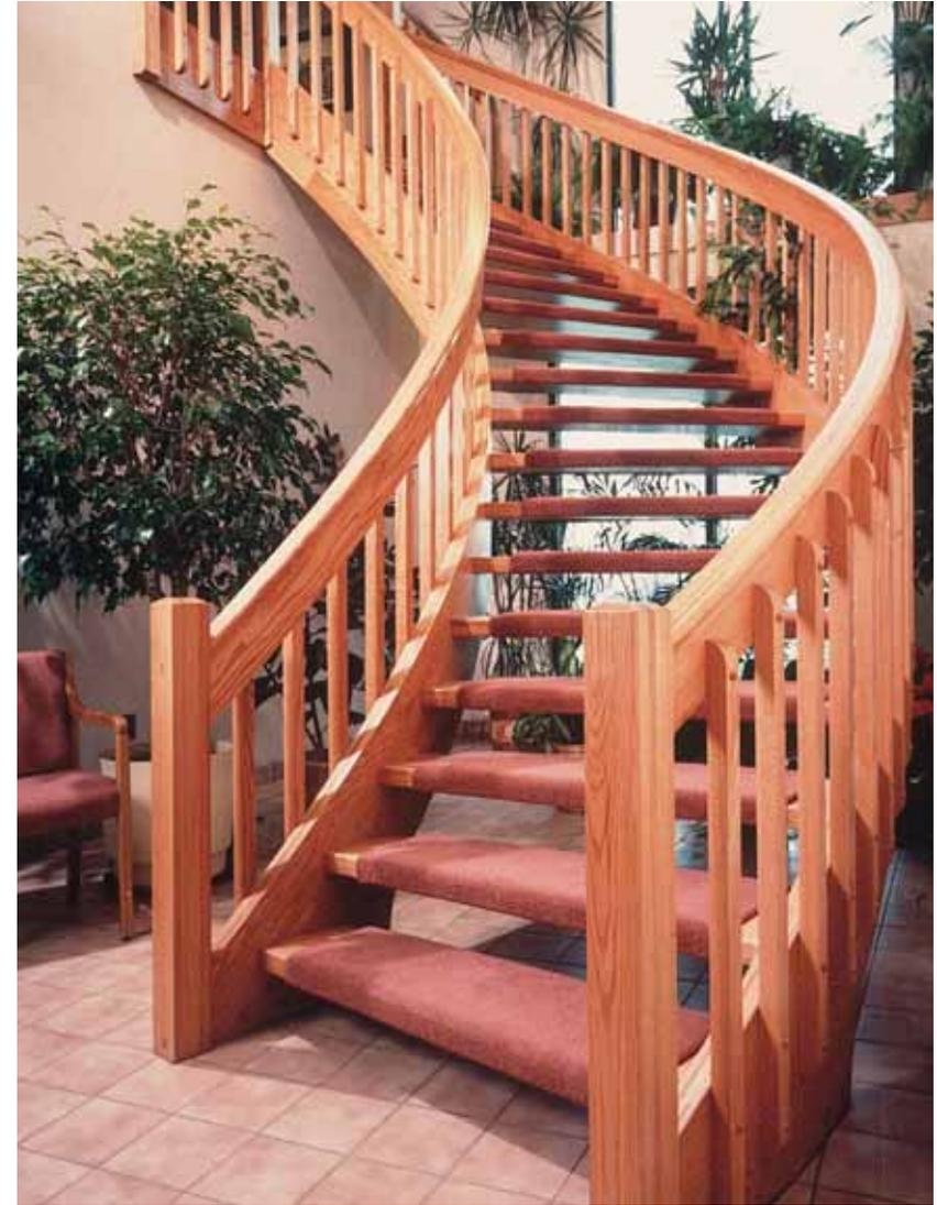
This freestanding curved stair was completely fabricated in a manufacturing plant and then disassembled and shipped to the building site. (L.J. Smith, Inc.)
