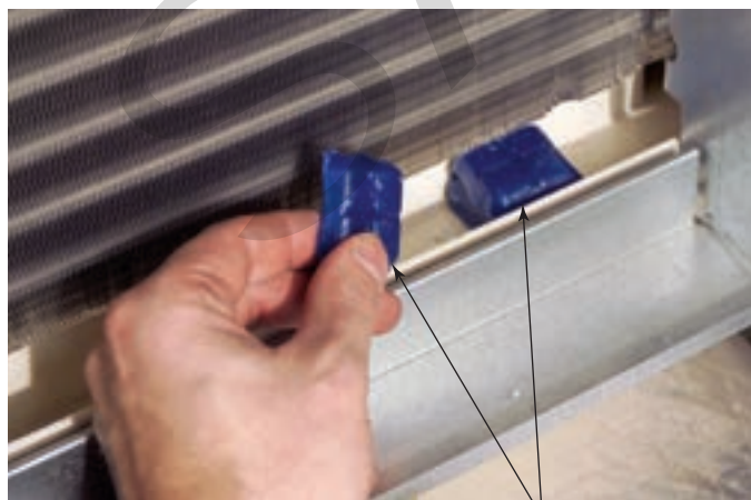
Figure 23-44. Placing algaecide tablets in the condensate drain pan.
