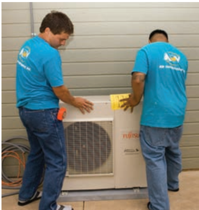
Figure 23-59. Two technicians positioning an outdoor unit on a mounting pad.
