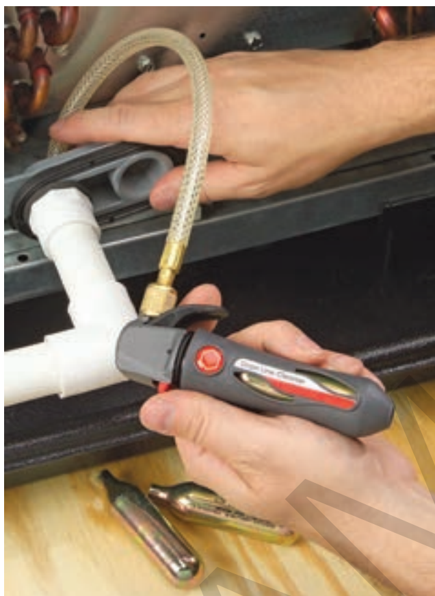
Figure 23-43. This drain cleaning gun blows away drain blockages using dry, compressed carbon dioxide.
