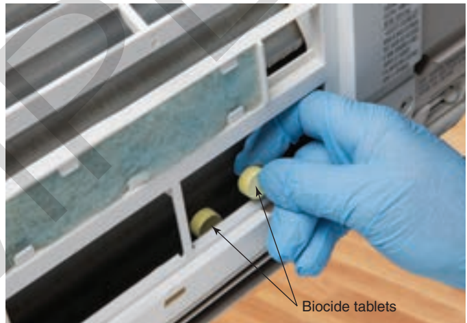
Figure 23-63. Adding biocide tablets to an indoor unit's condensate pan is often included as part of the unit's maintenance.
