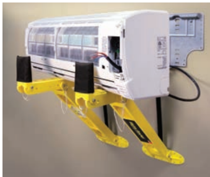
Figure 23-61. This wall bracket allows an indoor unit to be securely held in place while connections are made.
