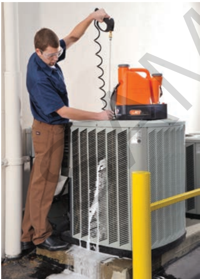
Figure 23-42. This technician is using a pressurized mix of chemicals and water flowing outward through the condenser coils.
