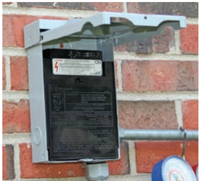
Figure 23-31. Electrical disconnect box. Note that the pullout contact can be pulled out or flipped upside down to disconnect the condensing unit so it can be serviced.
