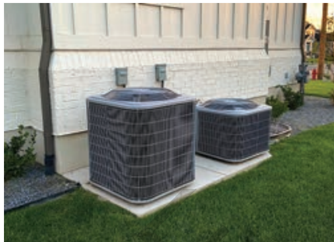
Figure 9-32. Two outdoor condensing units installed at a residence.
