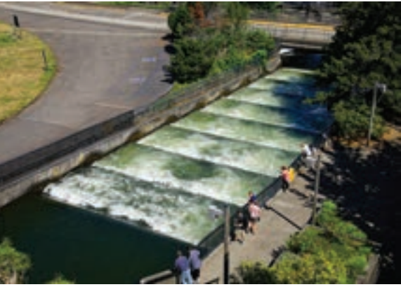
Figure 1-7. Fish ladders on the Columbia River at the Bonneville Dam in Oregon divert salmon from the dam and enable them to return upstream to spawn (lay eggs).
