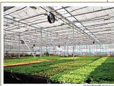
Figure 18-12. Framing for larger greenhouses can include steel trusses, I-beams, and other hardware for installed equipment, such as lighting. How are louvers or vents opened and closed in a greenhouse this large?
