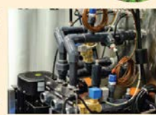
This reverse osmosis filtration system is used in a large, commercial greenhouse water system.
