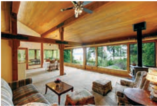
Figure 12-12. A residence making use of the post-and-beam system of framing.
