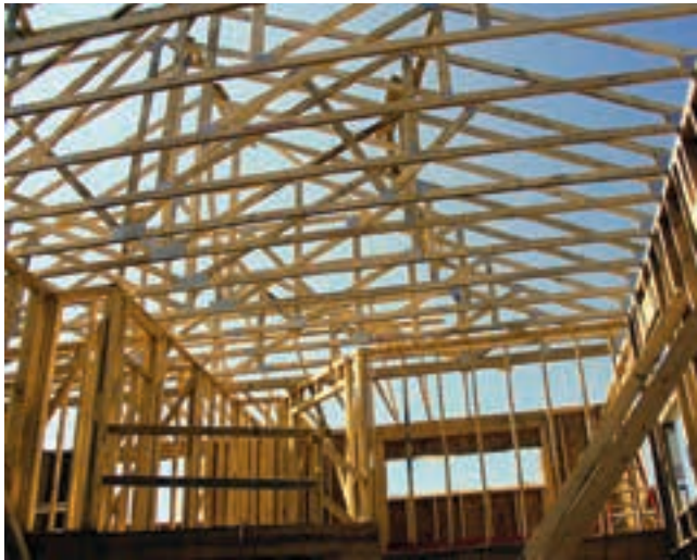
Figure 12-1. Wood is the most widely used framing material in residential construction, due to its flexibility and ease of use.
