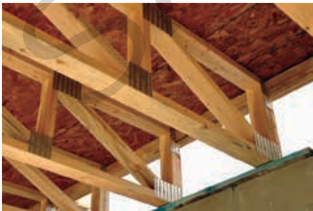
Figure 12-5. Open-web truss joists, also called floor trusses, are lightweight, high-strength members that have an open-web framework. The floor trusses shown have a web fabricated from wood members.
