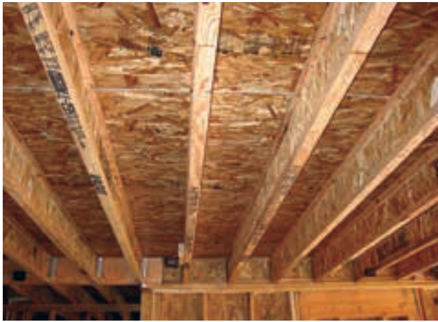
Figure 12-4. Wood I-joists are lightweight, high-strength framing members used for long spans. Common depths range from 9 1/2" to 16" and flange widths vary from 1 1/2" to 3 1/2". Member lengths up to 66' are available.
