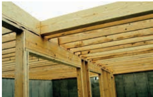
Figure 12-3. Wood floor joists framed over an interior loadbearing partition and foundation walls.
