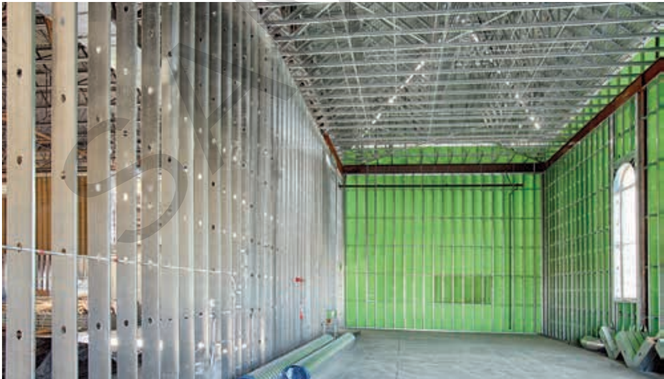
Figure 12-24. A variety of metal framing components is used in this commercial building project. Although residential use continues to grow, most metal framing today is used in commercial buildings.
