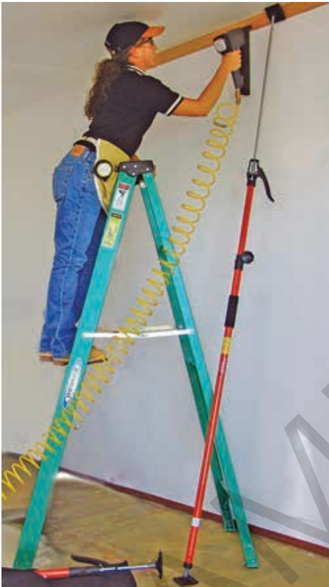
Figure 48-28. Support poles can be made or purchased. They help hold the crown moulding when working alone.
