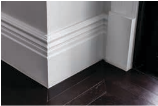
Figure 48-18. A plinth block at the base of this door provides a way for the base moulding to terminate nicely.
