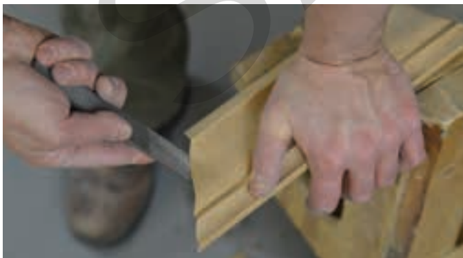
Figure 48-12. Coping crown moulding. A—Follow the edge of the face miter, angling the saw back from the face. B—Fine-tune the fit with a rasp.
