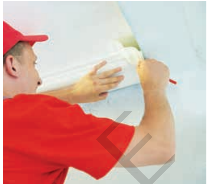
Figure 48-27. Using a short length of coped moulding to check the fit of an inside corner.
