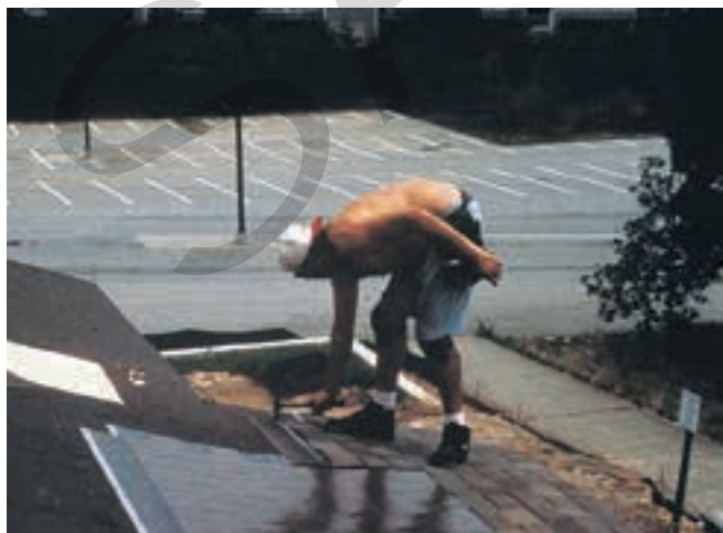
Figure 4.11 The Southface Eco Office and Resource Center buildings have many innovative features for offices and homes (A). Photovoltaic shingles are installed on the roof of the Southface Resource Center to make electricity from the sun's rays (B). The "light shelf" in the window area helps deliver the sunlight deep into this office space (C).
