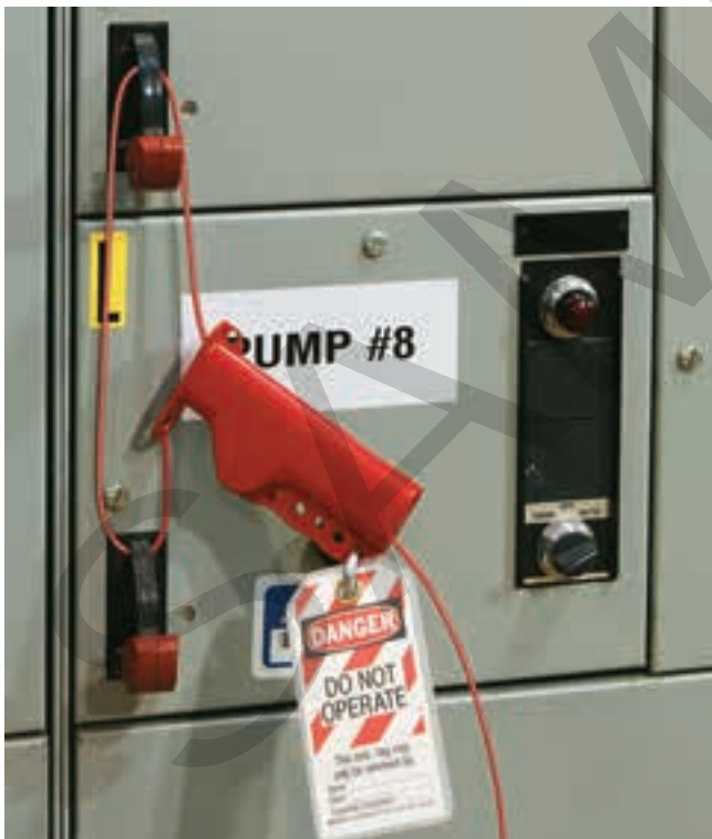
Figure 20-3. Work on de-energized equipment whenever possible. Always follow proper lockout/tagout procedures.
