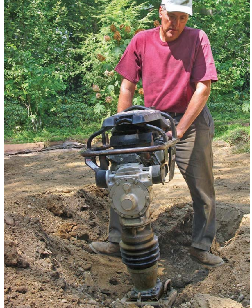
Small gas engines are used in a wide range of construction equipment, such as this power tamper. (Christina Richards/Shutterstock)
