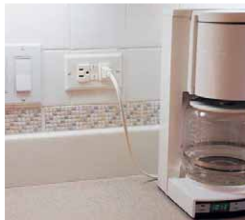
8-6 Electrical outlets with three holes indicate that an equipment grounding wire has been installed in the home. The two buttons in the center of this outlet indicate this is a GFCI.
